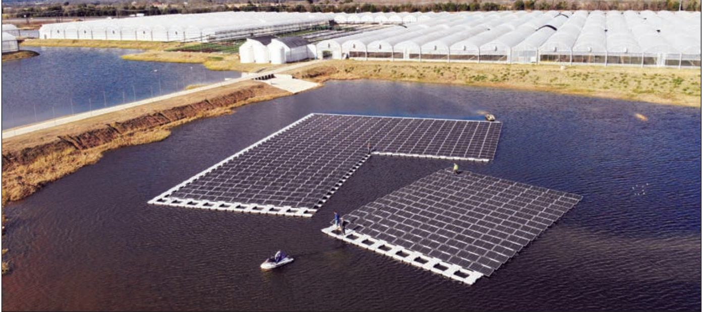
During installation, workers use personal watercrafts to maneuver parts of the array into position. Photo courtesy of Speir Commercial & Industrial
