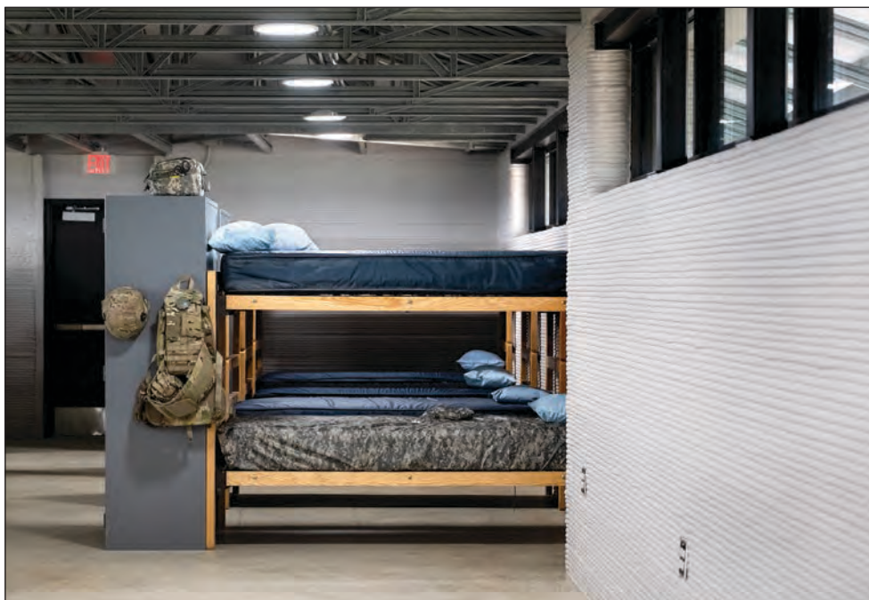
Above, a look inside the completed 3D-printed barracks to house Army or National Guard members for training at the military camp. Laura Skelding photo
