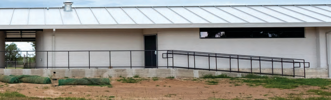
The largest 3D-printed building in North America is a 3,800-square-foot barracks that can house 72 military personnel at Bastrop County's Camp Swift. The computer-guided machine that built the barracks was developed by Austin-based company ICON. Laura Skelding photo
