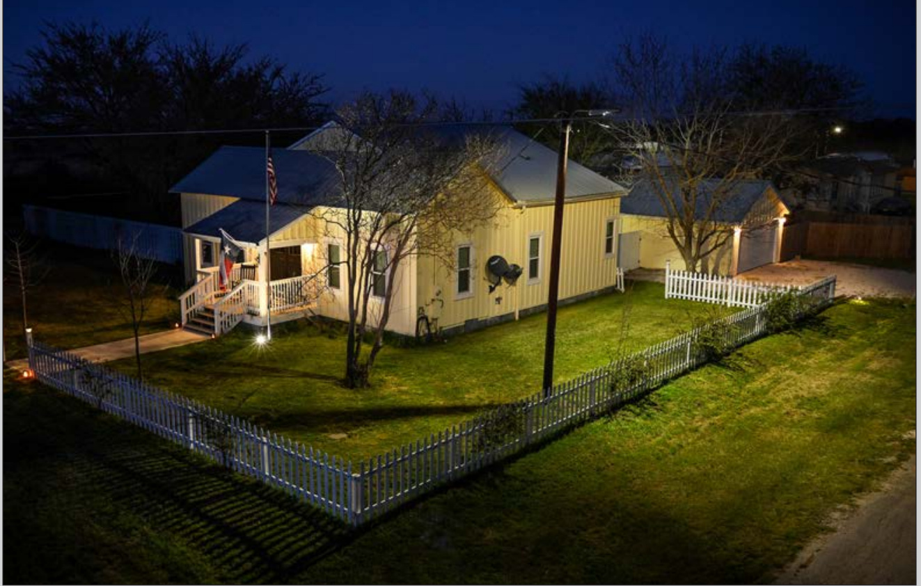
A dark-sky compliant security light illuminates a Bluebonnet member's property in Paige. Bluebonnet installs lights that shine downward but are shielded on the sides and top to prevent light pollution. Photo by Sarah Beal
