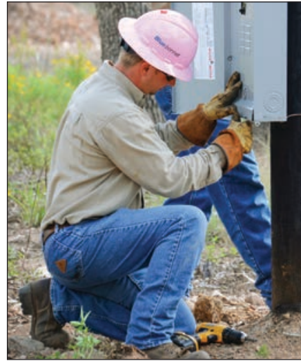
Logan Lancaster, a Bluebonnet crew supervisor from Giddings, left, installs a meter loop on a new pole while wearing a pink hardhat in support of Breast Cancer Awareness Month. All October, in addition to the pink hardhats and pink ribbon decals on trucks, Bluebonnet's member service centers will be lit pink to raise awareness for the cause. Sarah Beal photos
